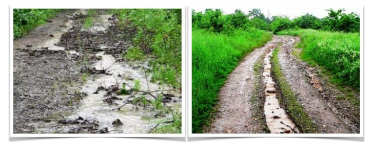
After the flood, waters carried the sediment away, depositing it downstream, eroding the road.
