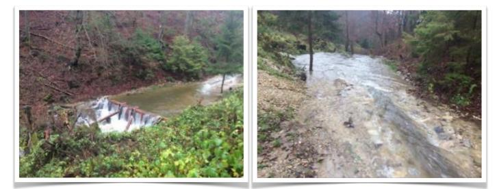
Log dam slows down the kinetic energy of the stream, preventing erosion. The height of the log dam allows fish to migrate. The picture on the right shows the same location upstream.
