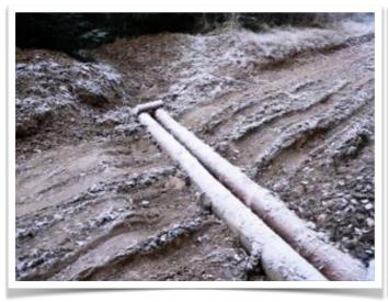
Intercepting cross dip and cross drain. Road drainage, utilizing a slope gradient.
