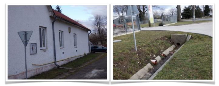
Draining rainwater in the township of Zemplínsky Klečenov (Trebišov). Concrete stream channel. Culvert. Unsustainable channelization and inadequate stream crossings alter hydrology and destroy aquatic life.
