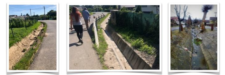
The old water paradigm at Kazimír, Malá Tŕňa (Trebišov district). The borough is discharging rainwater as an unnecessary resource. Impermeable surfaces seal the soil, reducing water infiltration, further dwindling groundwater supply.
