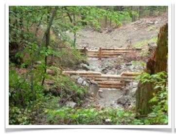
Log dams cascade repairing an erosion gully.
