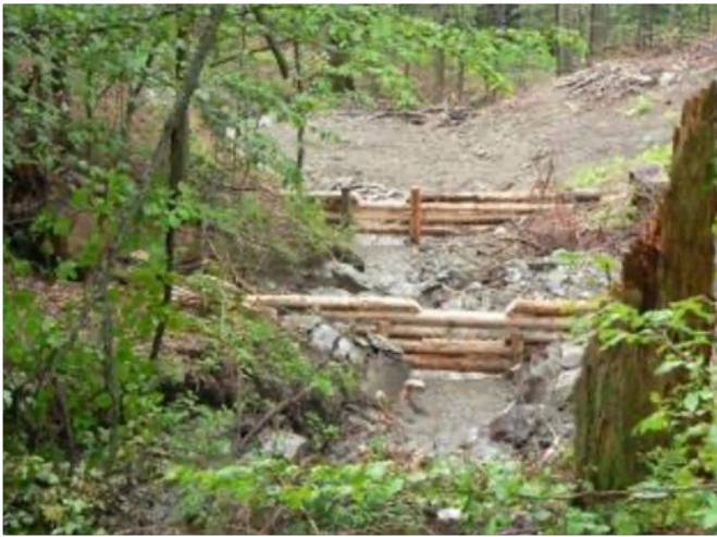
Log dams cascade repairing an erosion gully.
