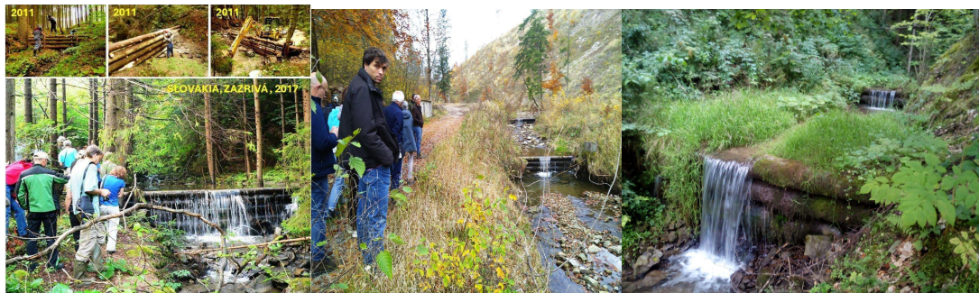
Figure 30 : On the stream, new wooden weirs in Hertnik ended stream narrowing in 2011. In 2018, the same weirs with alluvium moderated the water speed and stabilized the riverbed.
