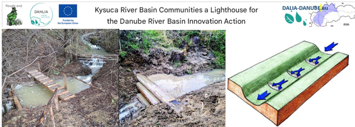
Figure 20 : Cascade of water retention measures on periodically drying up small watercourses
